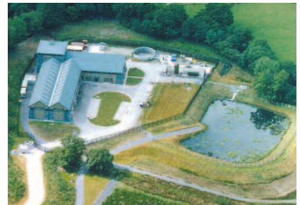
Example of remote pumping station.
