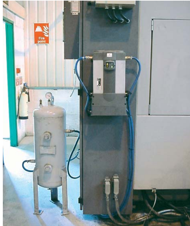
PNEUDRI MiDAS installed to supply control air for a CNC machining center
